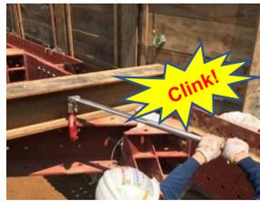
[Final tightening with the special torque wrench]
