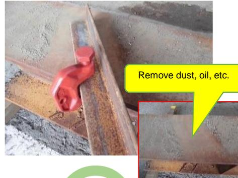
Dust and oil on a joining area must be removed. If foreign matters adhere to the area, the proof strength will decrease. Remove them before joining.
